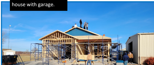
Students at SRCTC in Wahpeton built a house with garage.
